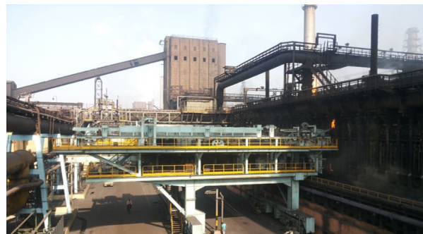
Heavy Engineering Corporation Limited, Ranchi, Jharkhand Photo: Hecltd.com
